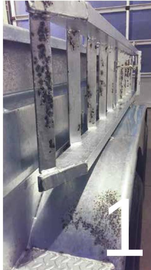
**Photo 1 :** Example of galvanized material exposed to de-icing salts before the natural passivation of zinc has taken place.
