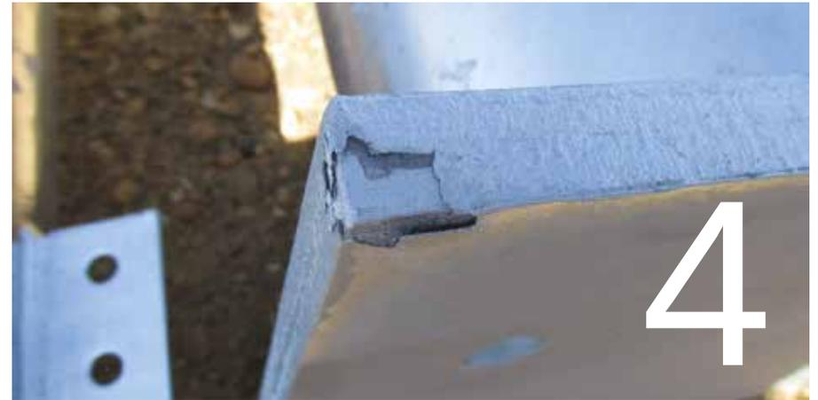
**Photo 4** : Example of galvanized material requiring repair.
